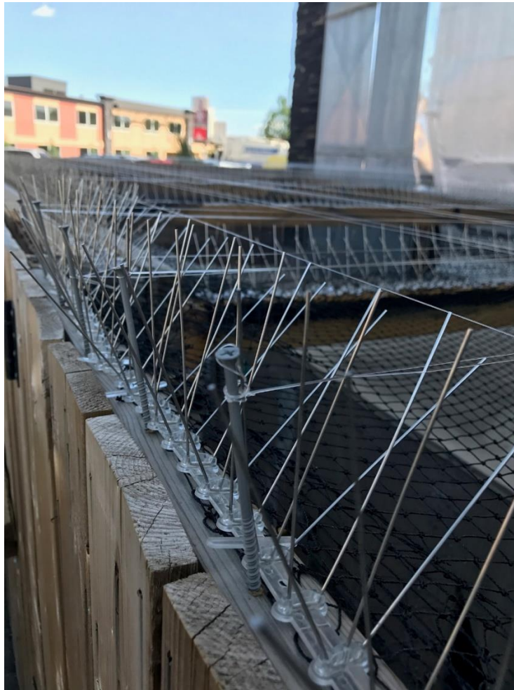
Photo 10: Closeup of spikes used to deter birds in urban roosting areas (Credit: Joro)
