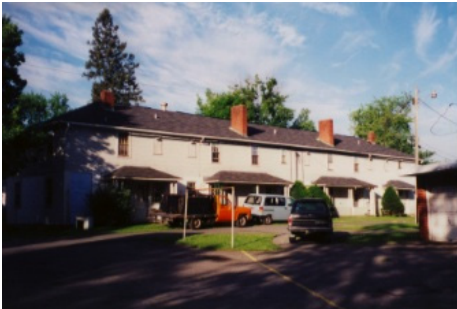
Figure 8.1. Faculty Court, which was demolished in 2000.
