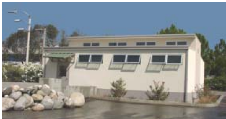
This modular relocatable structure is a prototype and contains a variety of high performance features such as daylighting, high indoor air quality, significant energy savings, and resource efficient materials.
