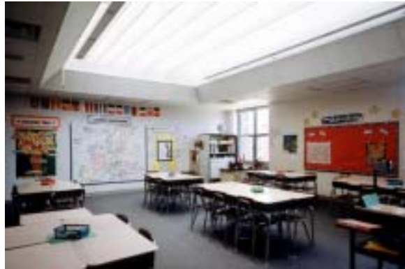
Toplighting reduces the glare and allows for a more even distribution of daylight within a space. NREL/PIX08834
