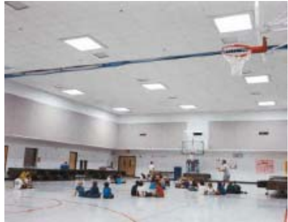
Grid of skylights provide even illumination across the space.
