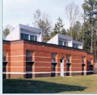
Figure S4.2 South-facing monitors.
