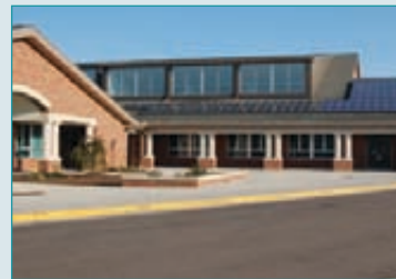
Figure S9.1. Clerestory windows and 24 kW PV system.
