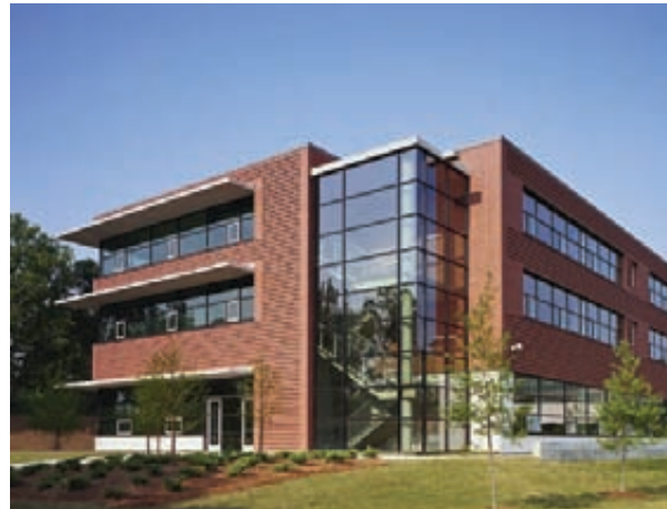
Figure 4.7. Building exterior with light shelves.
