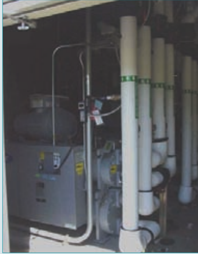
Figure S7.1. Water source heat pump.
