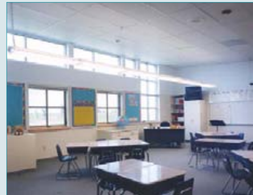
Figure S3.1. North-facing classroom with daylighting and sloped ceilings.
