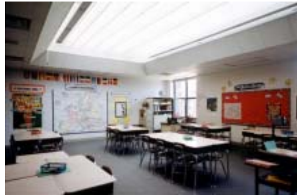
Toplighting reduces glare and allows for a more even distribution of daylight within a space. NREL/PIX 08834
