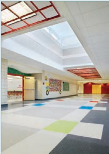
Figure S2.1. Corridor daylighting.
