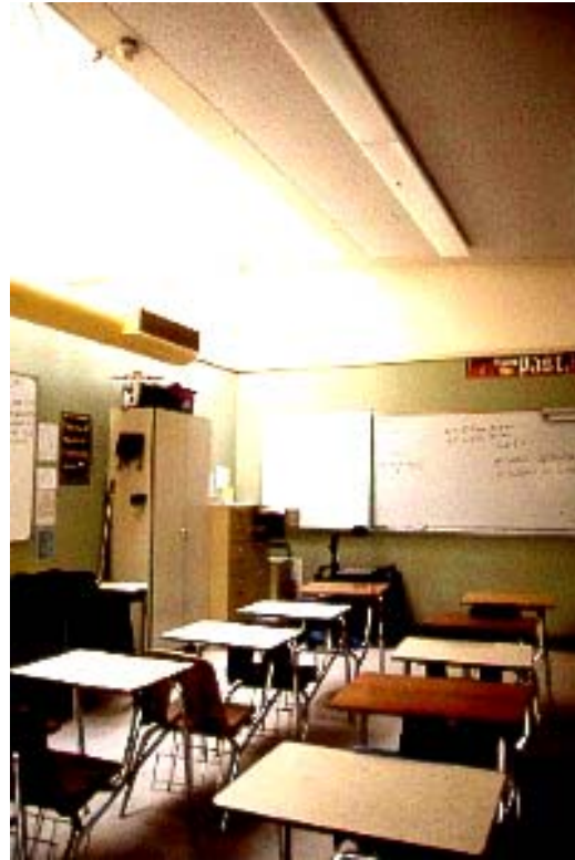
Skylit wall wash delivers daylight across two-thirds of this classroom.
