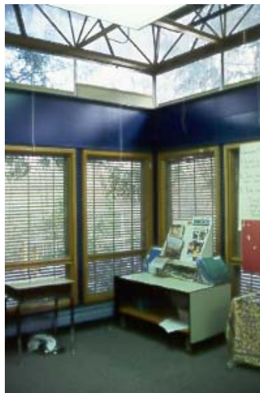
Horizontal blinds allow control of brightness from lower view windows. Note that high clerestory windows have no blinds so that daylight can reach deep into classroom. Most classrooms do not need complete black out capability for viewing of modern video equipment.
