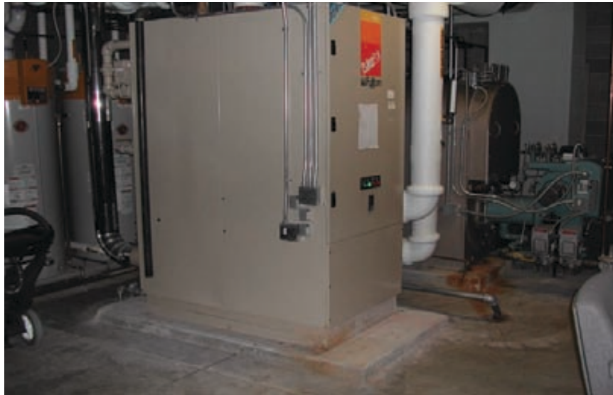
Figure 4.18. Pulse condensing boiler.
