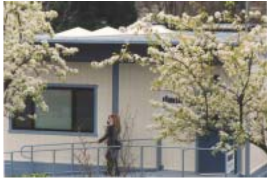
Pyramid skylights on experimental portable classroom design integrate skylights into a high efficiency modular design. NREL/PIX 11400
