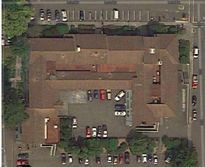
Figure 2.1: Building Arial View (source: google.com)
