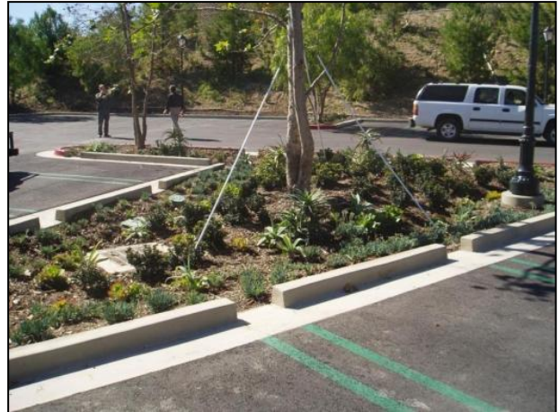
Bioretention in a Parking Lot
