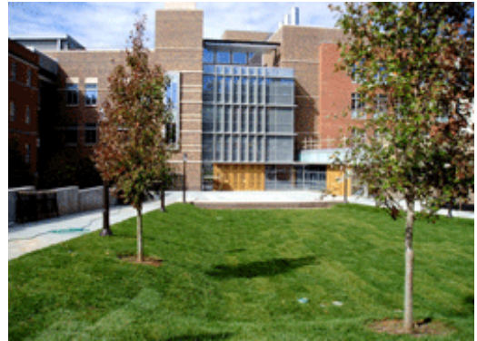
Use of varying color and glass mark the entrance to the building
