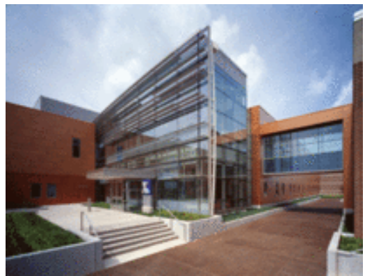
Transparency, change of material and raised plaza mark building entry, Harper College
