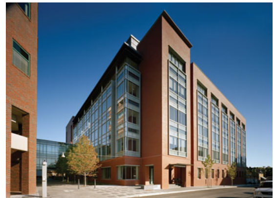
Curtain wall unifies, vertically, the floors of the building, Brown University
