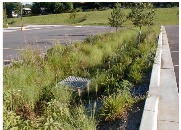
Bio-retention area in parking lot
