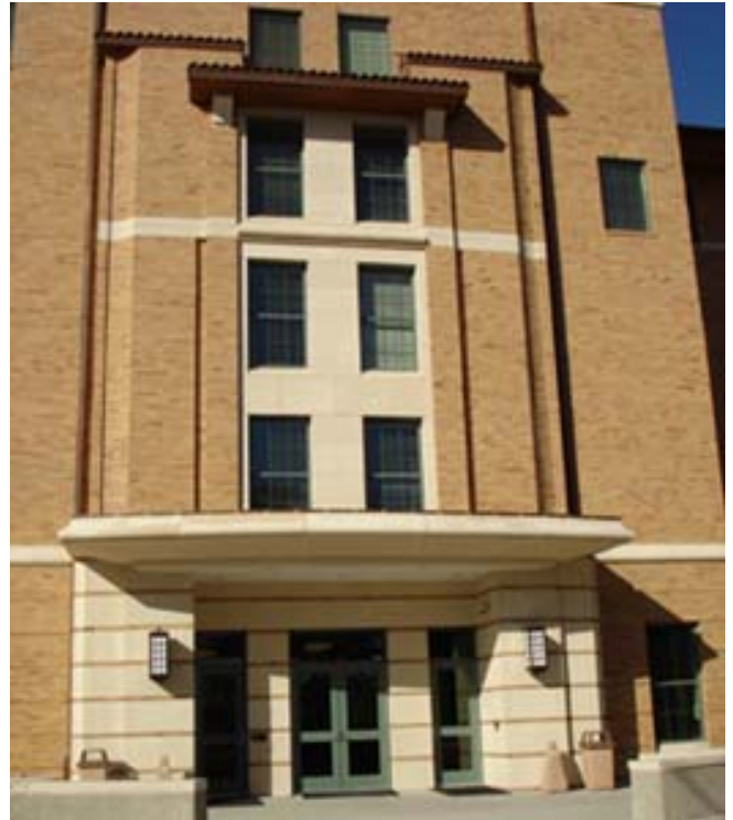
Use of masonry, stone and overhang to emphasize building entry, University of Texas - Austin
