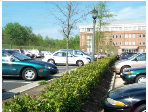
Bio-retention area in parking lot
