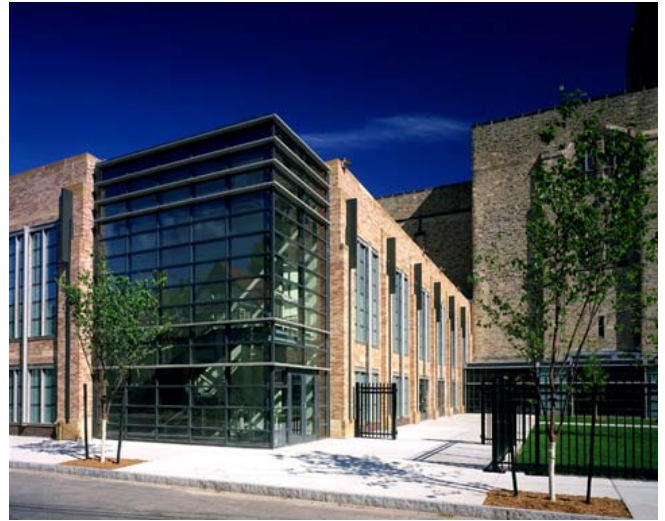
Use of curtain wall provides for rhythm, scale and transparency, Yale University
