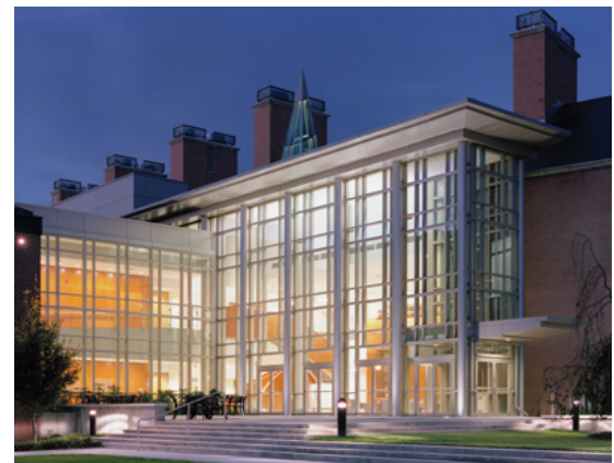
Pattern of the curtain wall system provides sense of scale at entry. Transparency gives the building depth, Gettysburg College.
