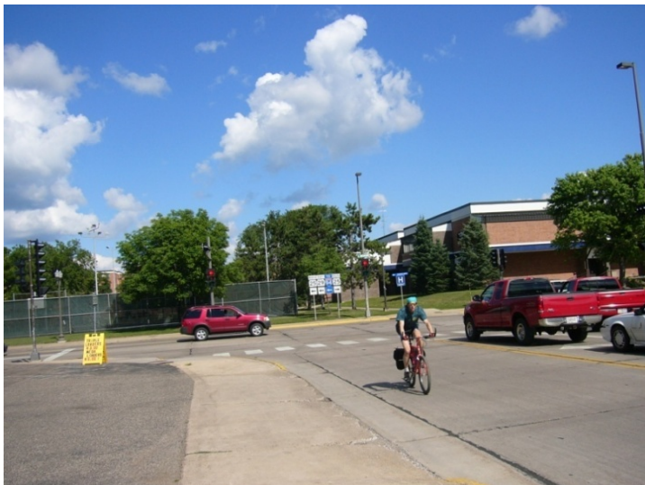
STH 29 and Broadway Intersection Looking East
