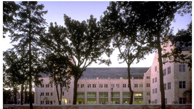
Background Building – St. Thomas University
