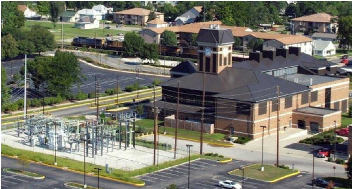
Figure 8: The natural gas fired Central Steam Plant constructed in 2001.
