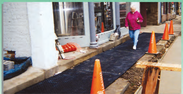
VersaMATS lock together to form continuous walkway
