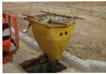
Removed Siltsack® is now ready for cleanout.
