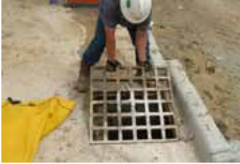
Remove grate from catch basin.
