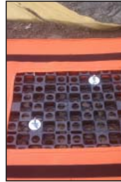
Install base with 2 to 4 anchors as needed.
