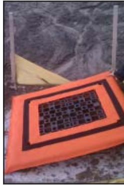
Install Grate Pyramid base over grate.
