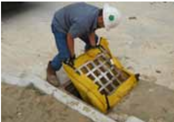
Replace Siltsack® and grate inlet into recess.
