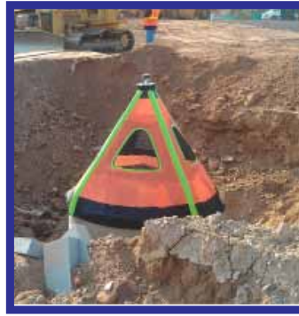
Type B - for riser pipe installation
