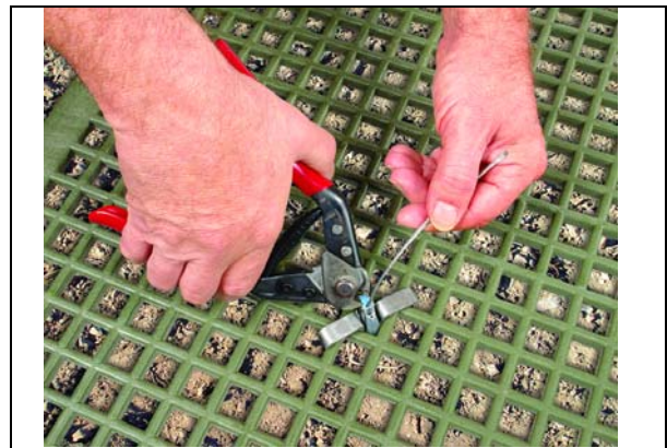
Figure 10. Cut the cable flush with the Gripple
