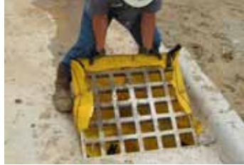
Slide Siltsack® over one side of grate.
