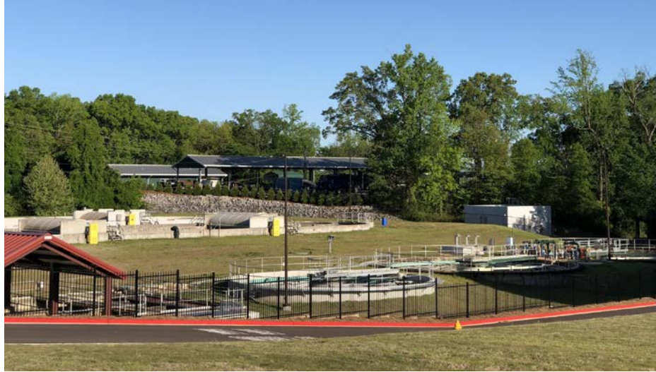
Figure 9. University of Mississippi wastewater treatment plant.
