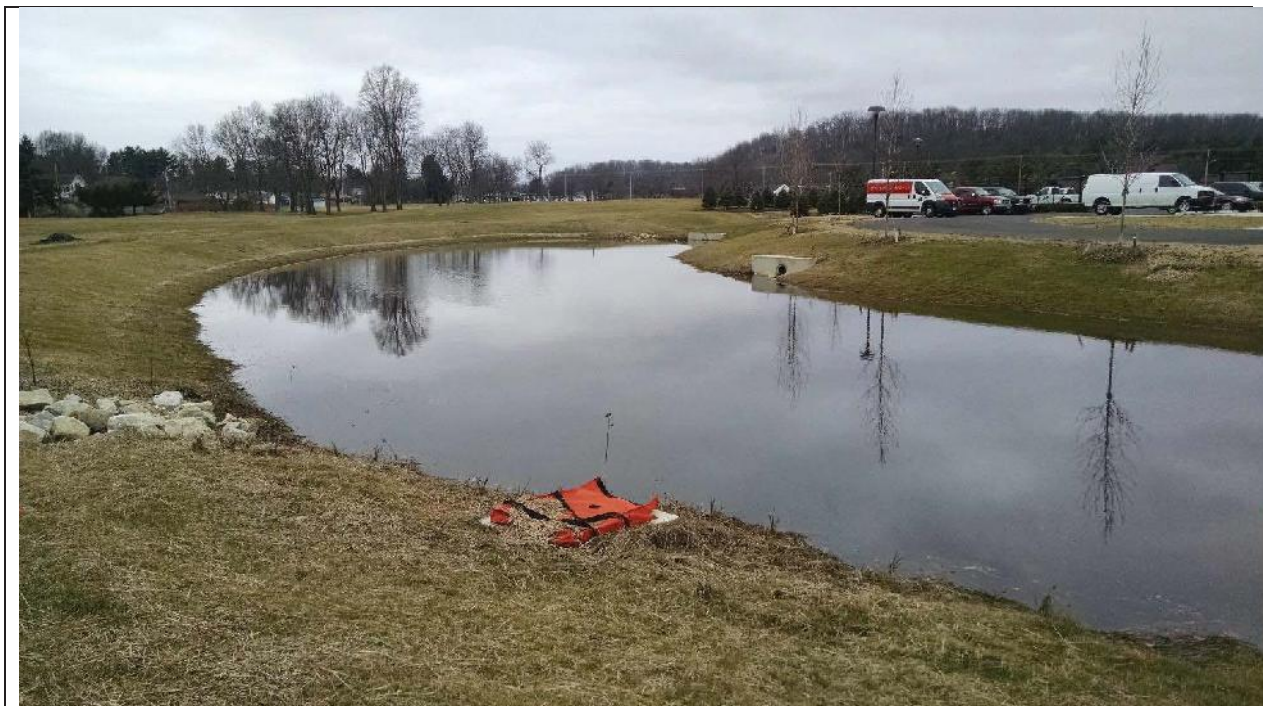
Stormwater Infiltration Basin
