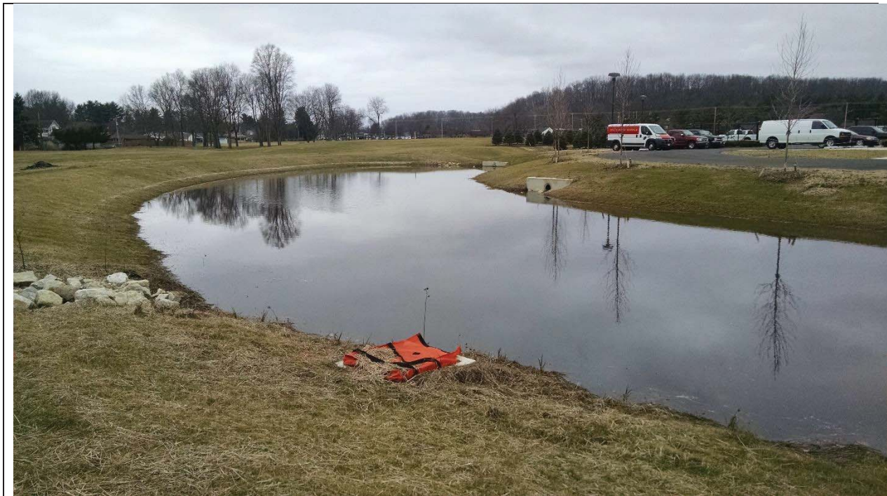
Stormwater Infiltration Basin
