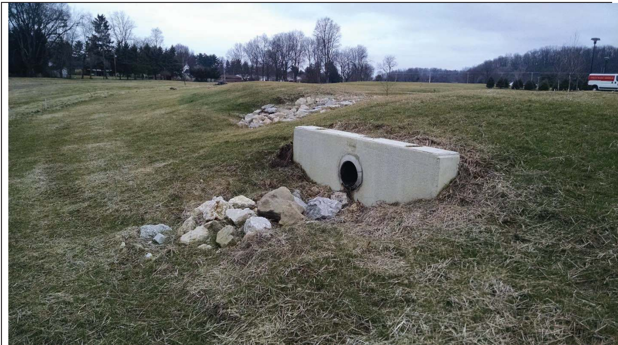
Stormwater Infiltration Basin – Facility Outfall
