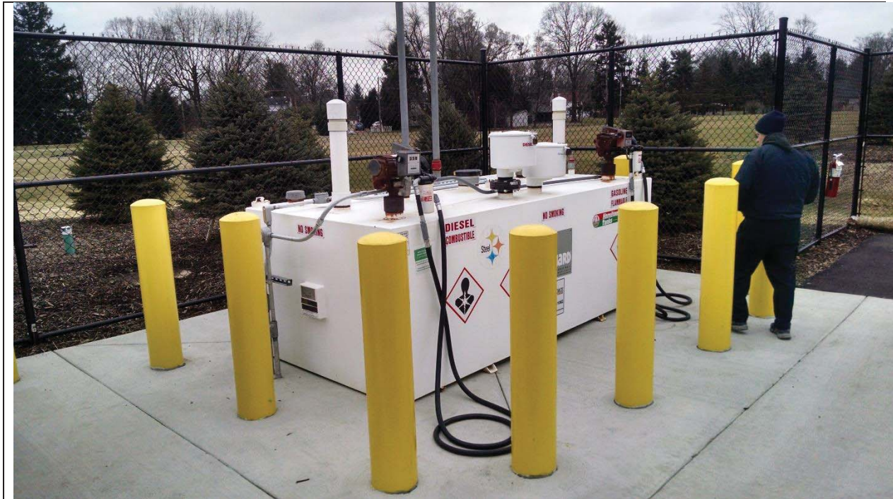
Fuel Pump Station
