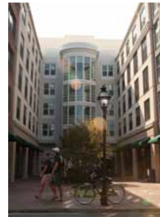
George Street Apartments
