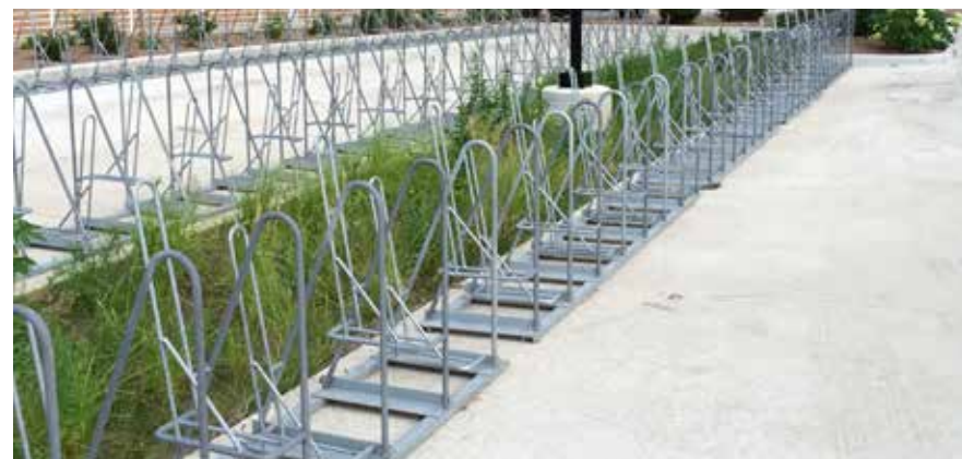
Figure 5-38 Infiltration Planter Between Bike Racks, Wis. Institute for Medical Research
