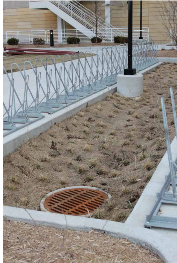
Figure 3-17 Biofiltration area, Wisconsin Institute for Medical Research
