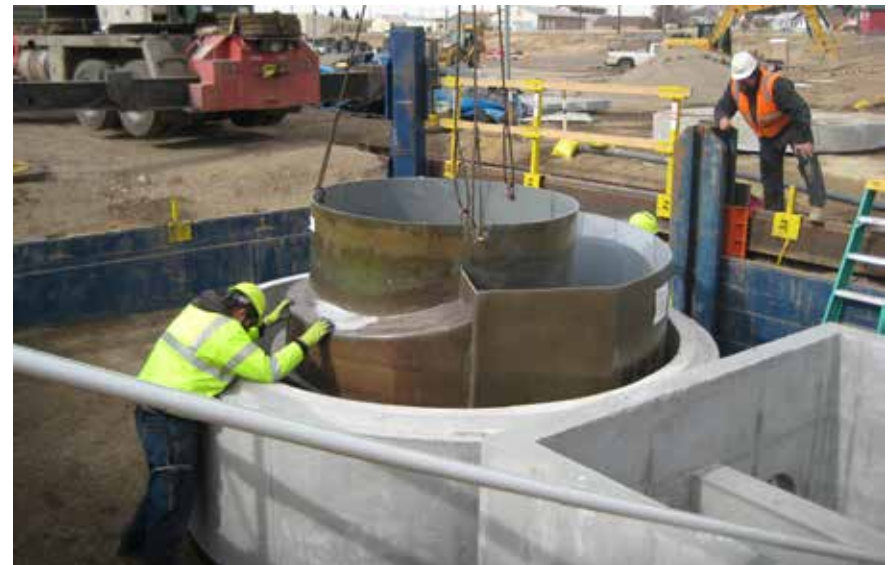
Figure 5-48 Installation of a Hydrodynamic Device, Butte, Montana
