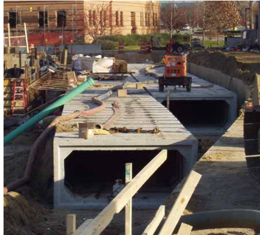
Figure 5-60 Utility Project on East Campus Mall
