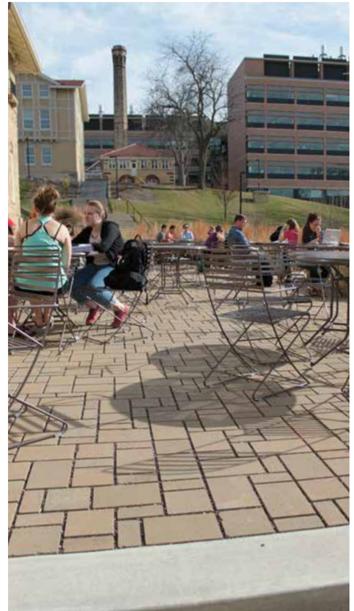
Figure 1-2 Permeable Pavement, Carson Gulley Commons
