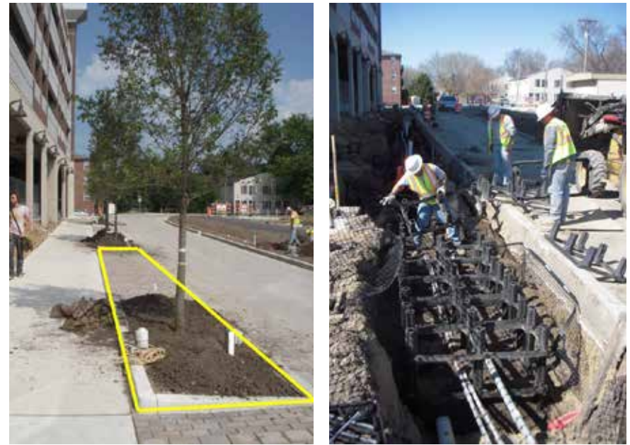
Figure 5-53 Installation of Silva Cell Root Enhancement Zone
