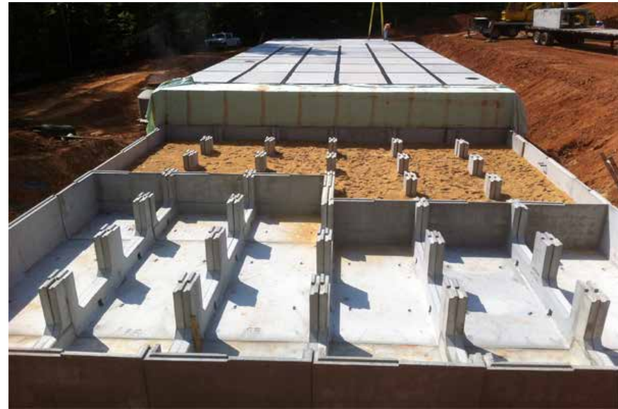
Figure 5-13 Underground Detention Precast Units Being Installed
