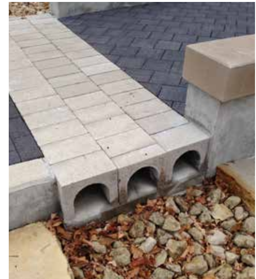
Figure 5-52 Modular Concrete Flume for Walks
