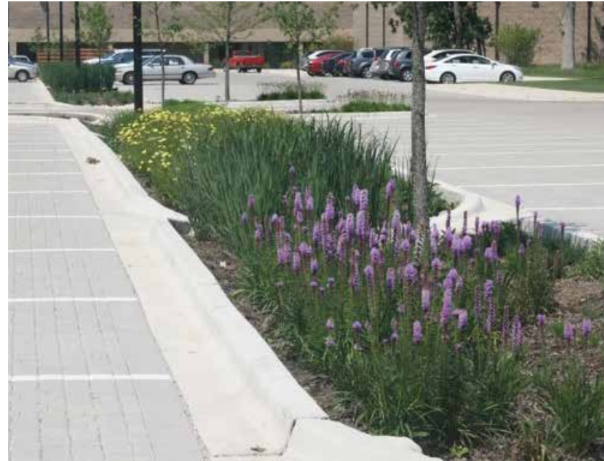
Figure 5-5 Parking Lot Median Bio Filters
