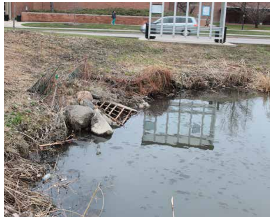
Figure 3-12 Nielsen Pond Stormwater Outfall
