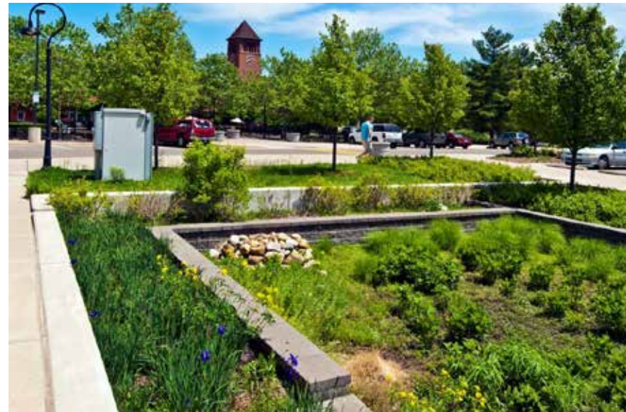
Figure 5-20 Biofiltration Area in Battle Creek, Michigan
