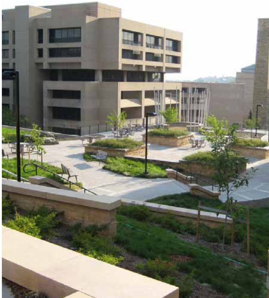
Figure 5-26 Education Building First Floor Green Roof (Over Parking)
