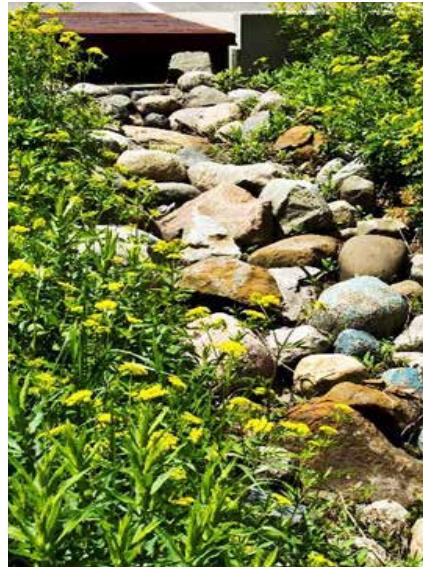
Figure 5-49 Stone Conveyance Channel
