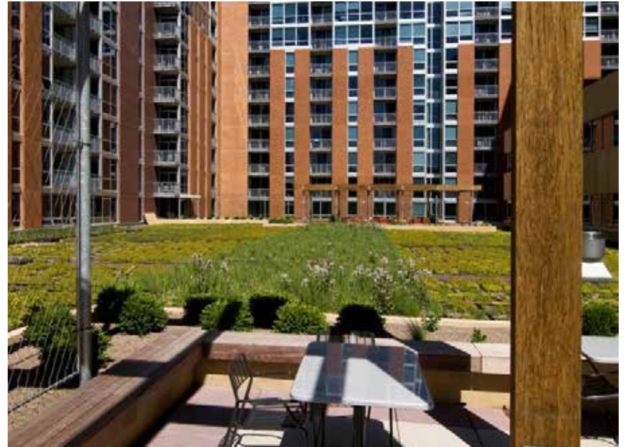
Figure 5-35 Green Roof, University Square
