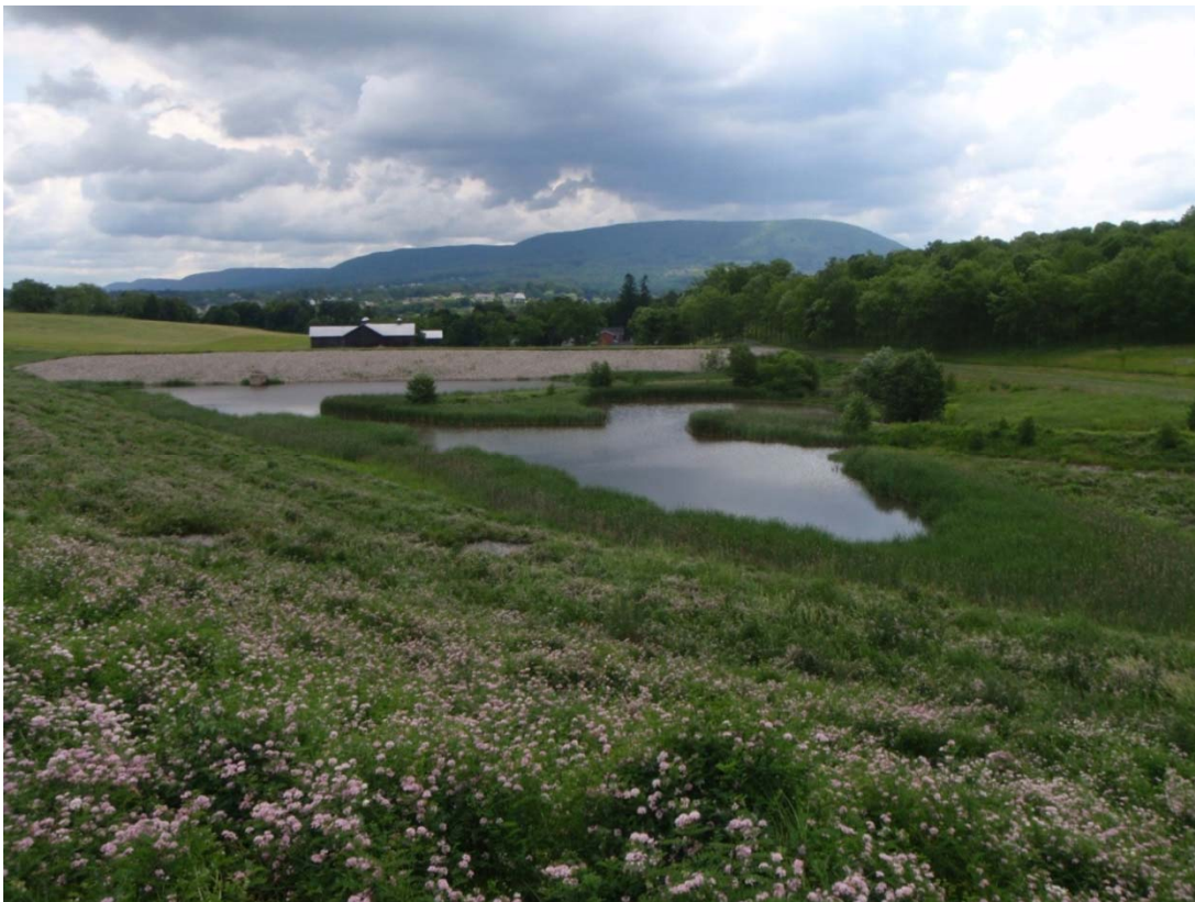
Figure 4.g. Bathgate Dam after 2000 Upgrades
