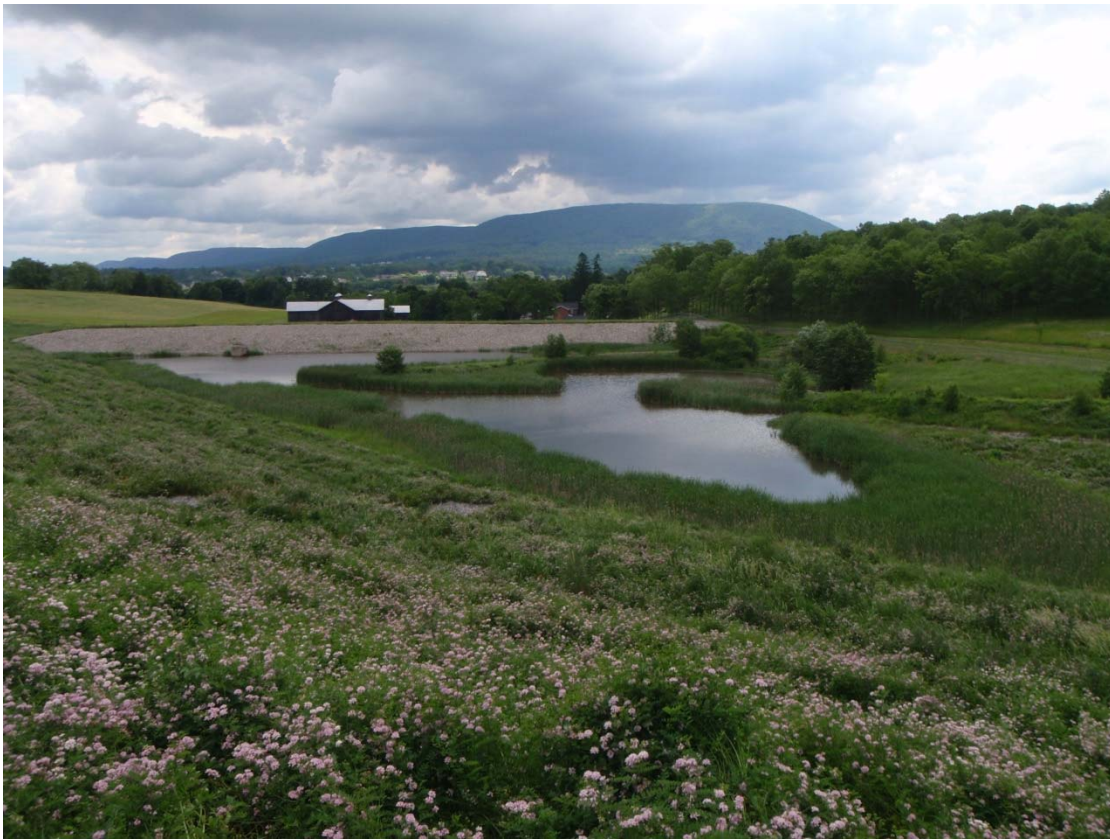
Figure 8.b. Bathgate Dam as seen from the Western Gate
