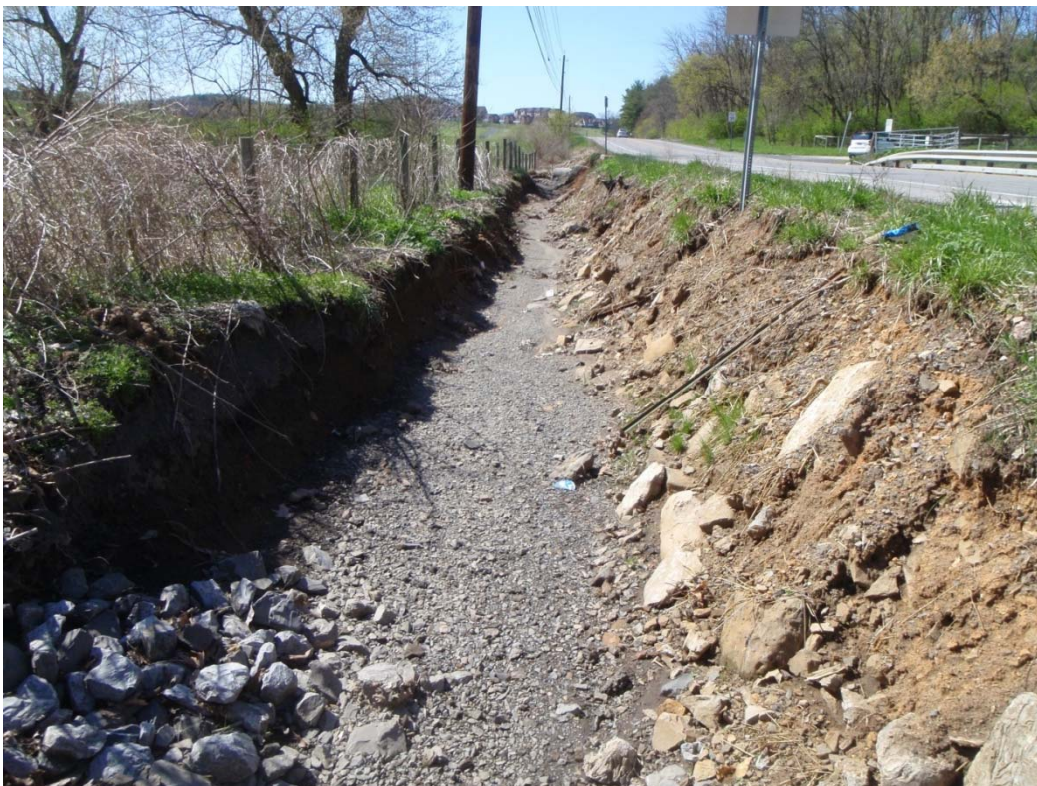
Figure 7.k. PennDOT Controlled Swales along Fox Hollow Road Section 7-10
