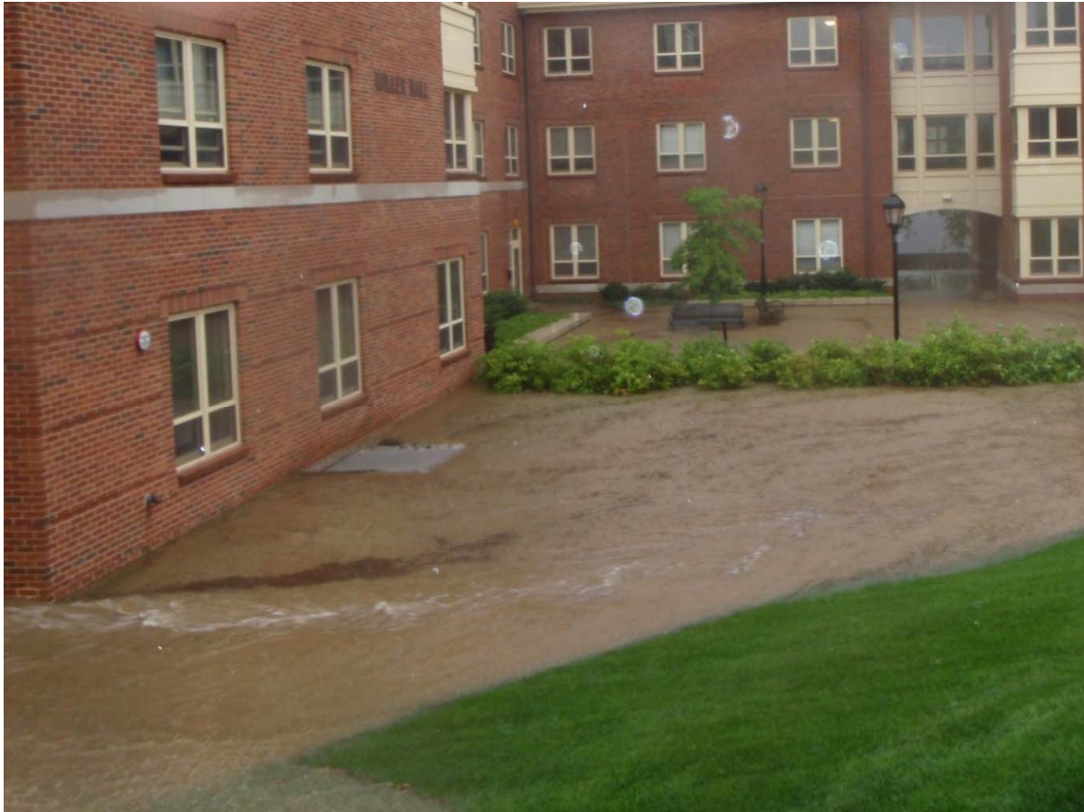
Figure 4.a. Example of Nuisance Flooding on Campus
