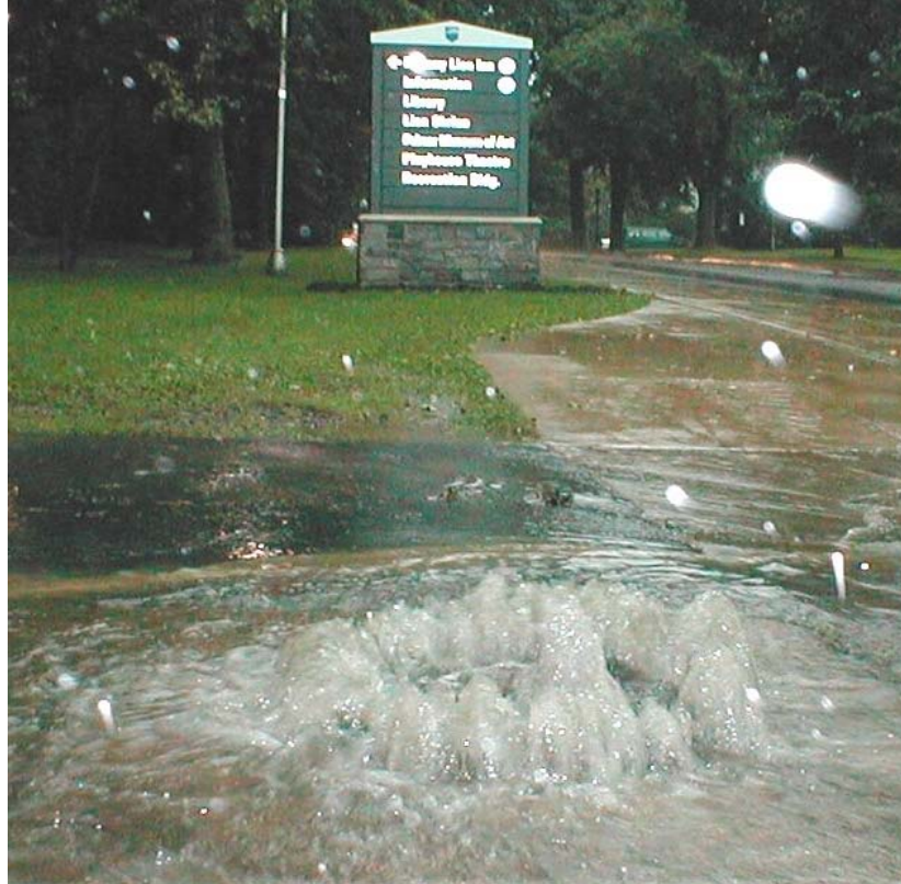
Figure 7.e. Surcharging at STMH125 along Park Avenue
