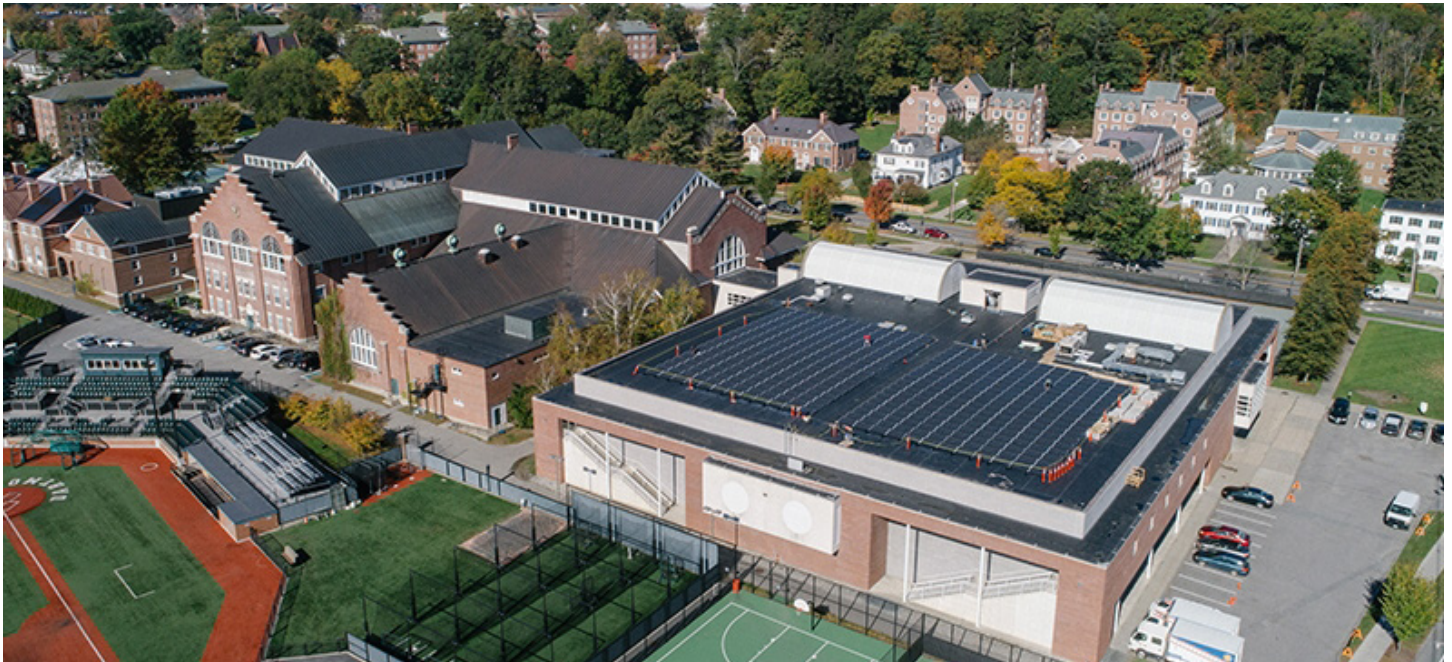
Solar panels on the roof of Berry Sports Center at Dartmouth College, installed in 2017
