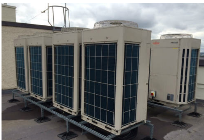
Variable refrigerant flow air-side unit
