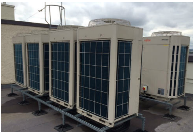
Variable refrigerant flow air-side unit
