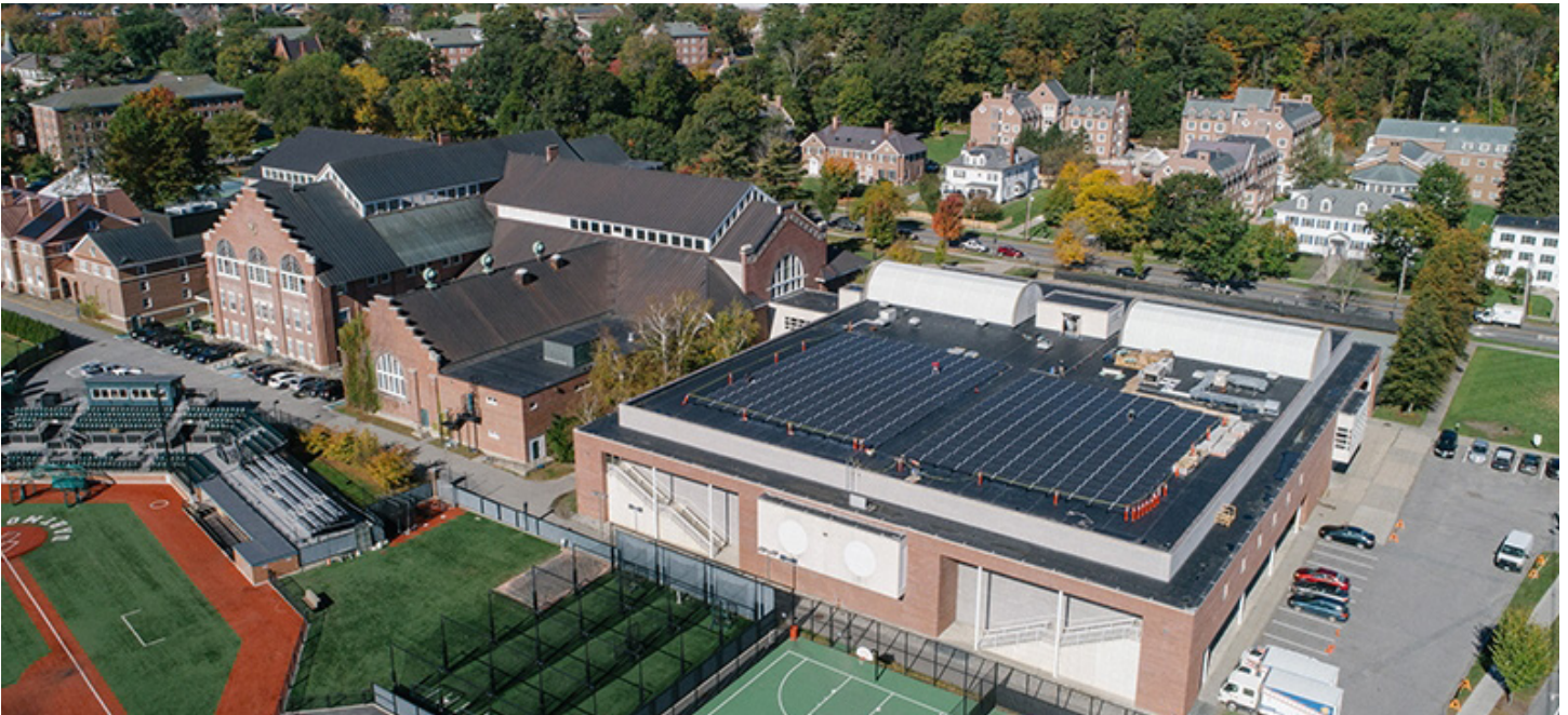
Solar panels on the roof of Berry Sports Center at Dartmouth College, installed in 2017
