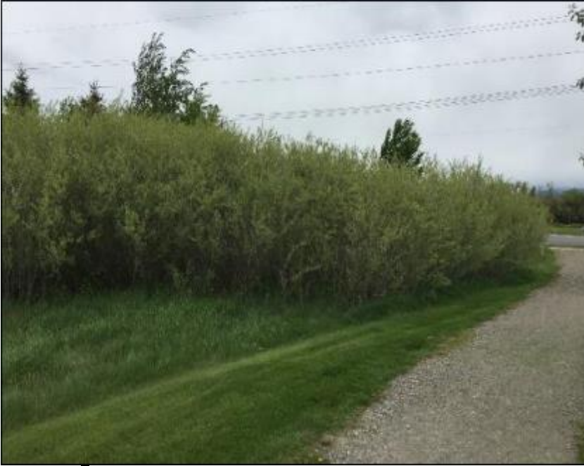
Image 6.0.1: Overgrown stormwater basin
