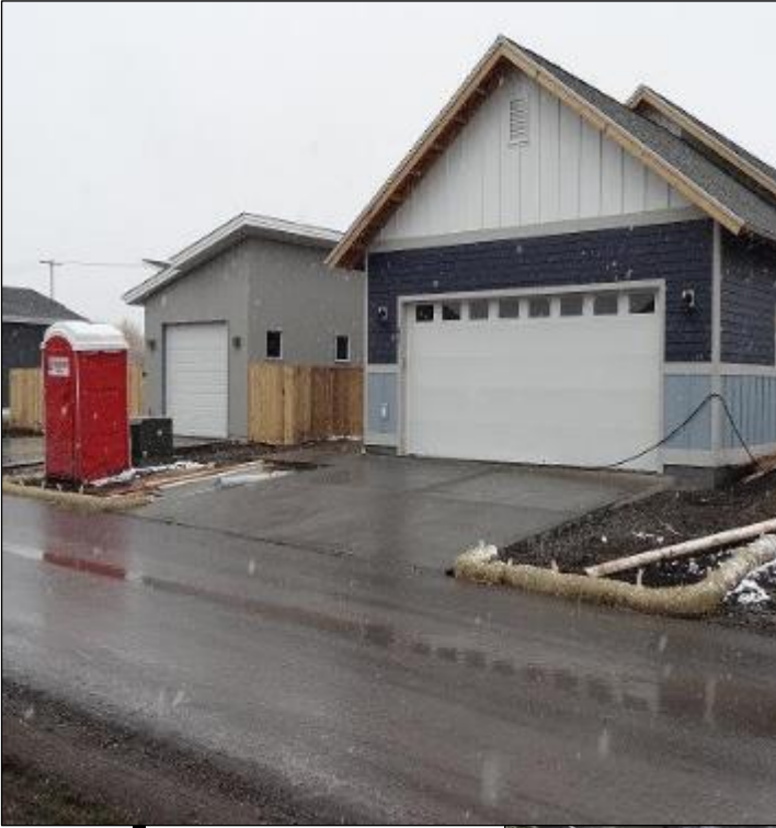
Image 5.0.1: Compliant single-family residential property
