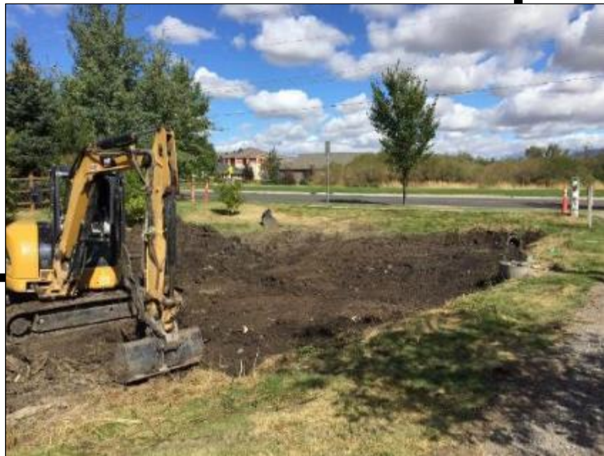
Image 6.0.1: Dredged stormwater basin
