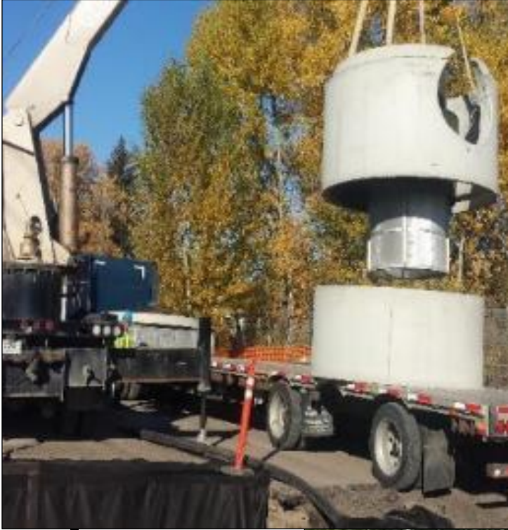
Image 2.0.1: Stormwater treatment unit installation
