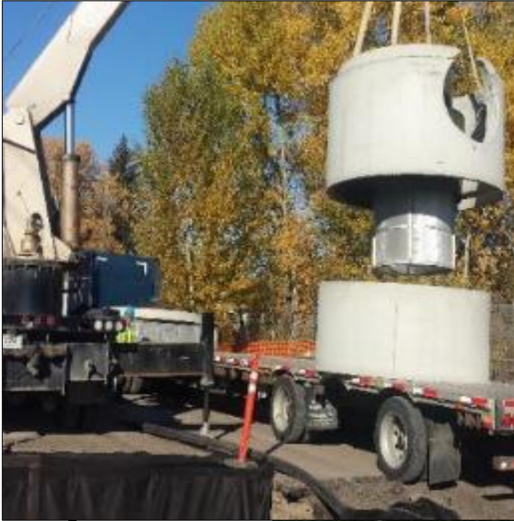
Graphic 2.0.1: Stormwater treatment unit installation
