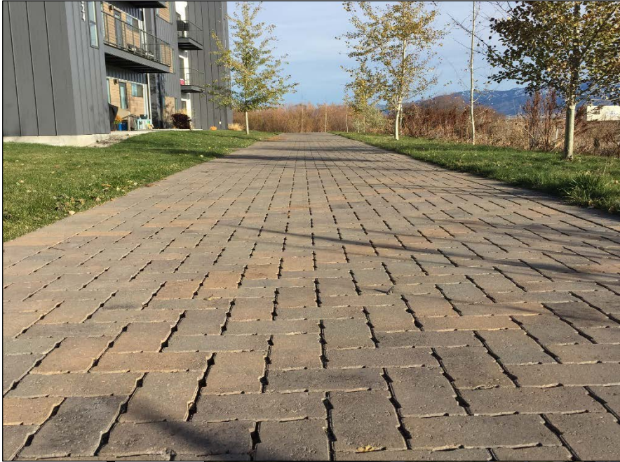
Graphic: 9.0.1: Permeable Paver Walkway
