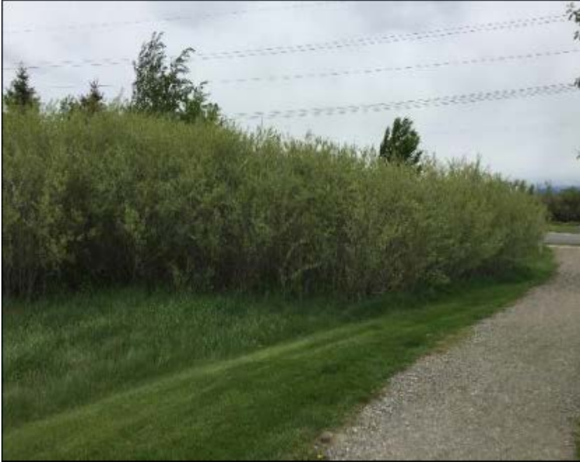
Graphic 6.0.1: Overgrown stormwater basin
