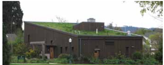
Many Nations Longhouse bioswale and green roof
