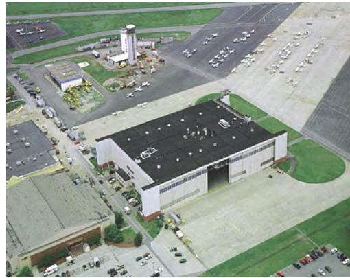
Hanscom Field Flight and Antenna Test Facility
