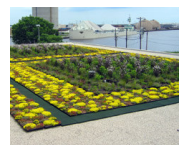
Great Lakes Water Institute Green Roof. Source: UW-Milwaukee
