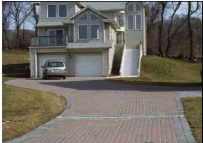
Figure 5.20 Permeable pavers as an alternative driveway surface
