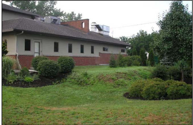
Figure 5.38 Rooftop disconnection for storage and infiltration, Guilderland, NY, NYSDEC
