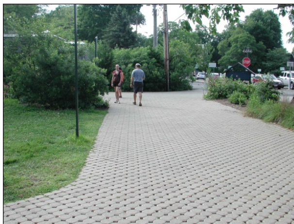
Figure 5.59 Walkway with permeable pavers -Scenic Hudson Park, Cold Spring, NY
