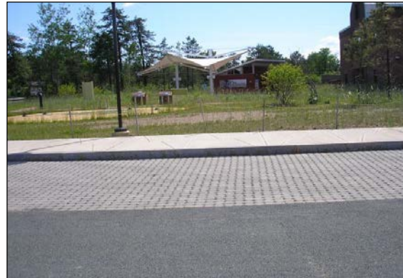
Figure 5.58 Asphalt, Permeable Pavers, Porous Concrete, Albany, NY
