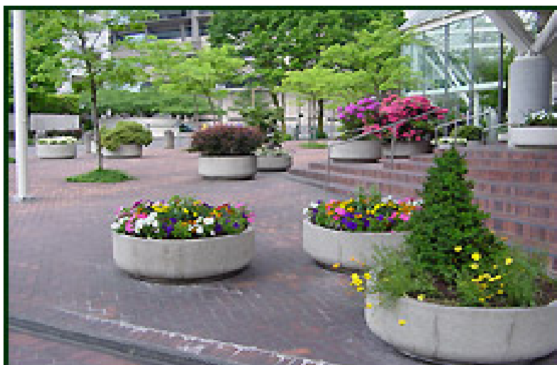
Figure 5.53 Contained stormwater planters made of concrete
