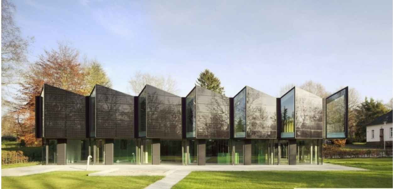
Figure IV.5. Building-integrated photovoltaics, such as on this day-care center in Germany, can be used on new campus buildings with PV displacing the cost of wall and roofing material.
