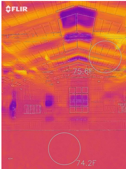
Figure 5.2.2 Thermal Images with VFD at 75% speed
