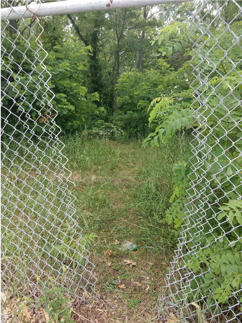
Figure 36: (North Campus Waypoint 6) Break in fence and informal pathway down towards the river. People were seen and heard along the embankment of the river.
