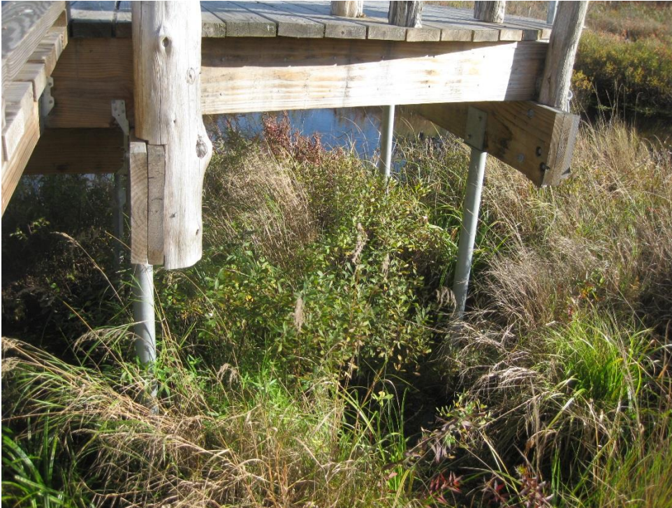
Figure 50: Vegetation growing under platform in Carlisle, Mass.
