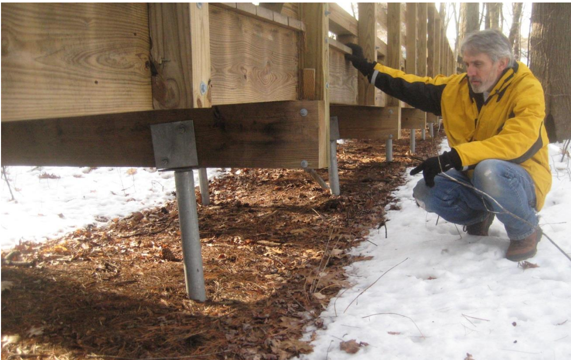
Figure 51: Helical piers in ground with minimal disturbance, Carlisle, Mass.
