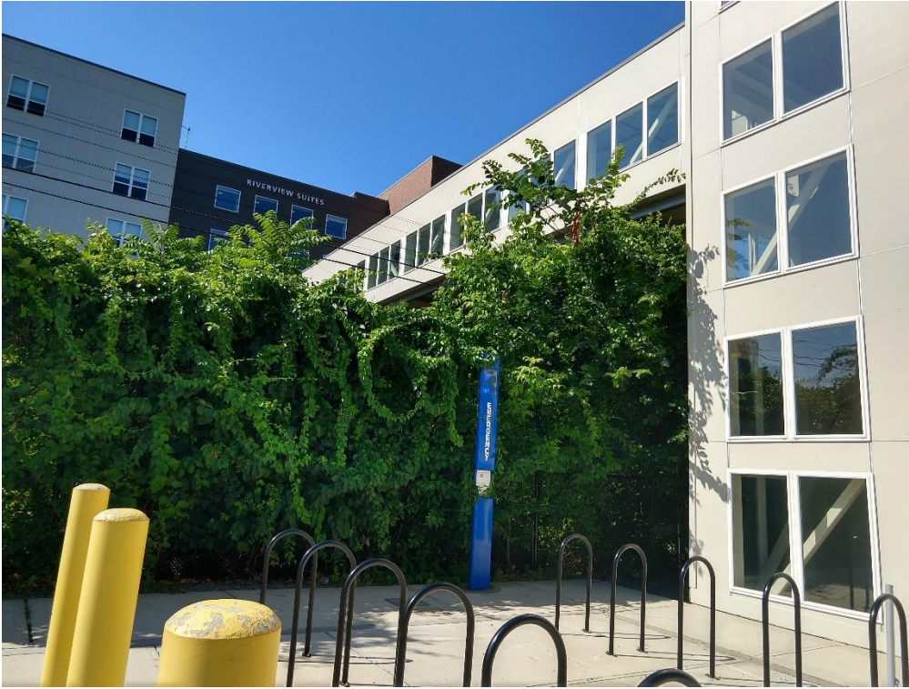
Figure 34 (South Campus Waypoint 2) Oriental Bittersweet growing on fence between Riverwalk Streets and catwalk. This area should be actively managed for invasive plants and restored with native berry producing shrubs. Students could watch wildlife foraging on the fruits from the catwalk.
