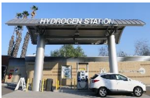
Cal State LA Hydrogen Station
