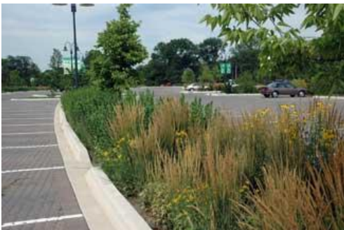
Bioswales located in a parking lot at the Morton Arboretum.
