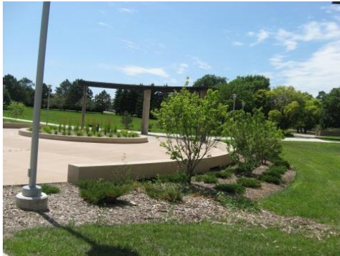
Poured in place concrete seat wall at Jackrabbit Village.
