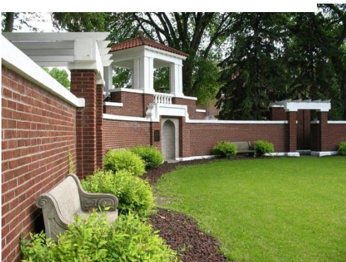
Sylvan Green located in the Historic District.
