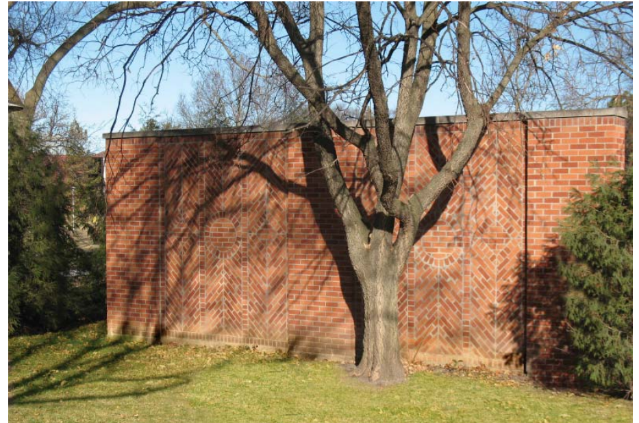
FIGURE 1.2: MASONRY SCREEN WALL (LINCOLN MUSIC CENTER)
