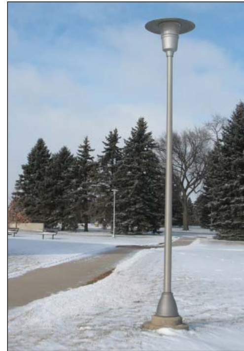
FIGURE 3.1: CAMPUS STANDARD PEDESTRIAN LIGHT FIXTURE
