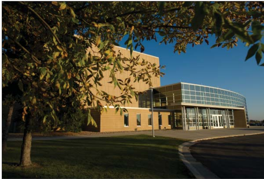
FIGURE 1.3: PERFORMING ARTS CENTER
