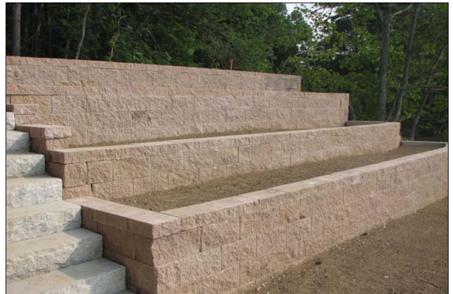
FIGURE 7.2: EXAMPLE – STRAIGHT-FACED UNIT RETAINING WALLS
