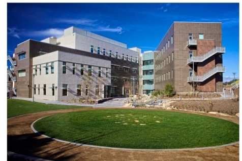
Social and Behavioral Sciences Building Opened Fall 2011 - LEED Silver Rating
