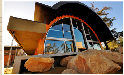
Architectural features, like the rain chain seen on the McMahan House, directs water in the ground
