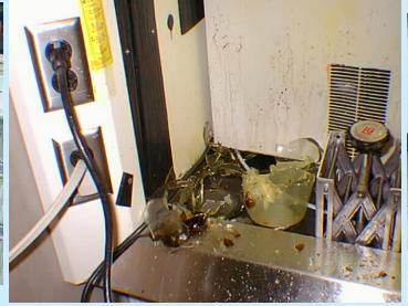
Improper chemical waste management caused this explosion and fire.
