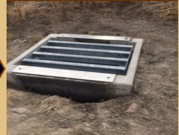
Sediment and overgrown vegetation around inlet has been removed. The screen and restriction plate holes have been cleaned out.
