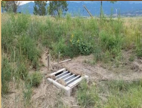
Outfall structure has been inundated with sediment from upstream erosion near Copper and Eldora House by Lot 230
