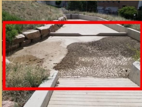
Significant build-up of sediment in sediment trap near Osborne Center for Science and Engineering
