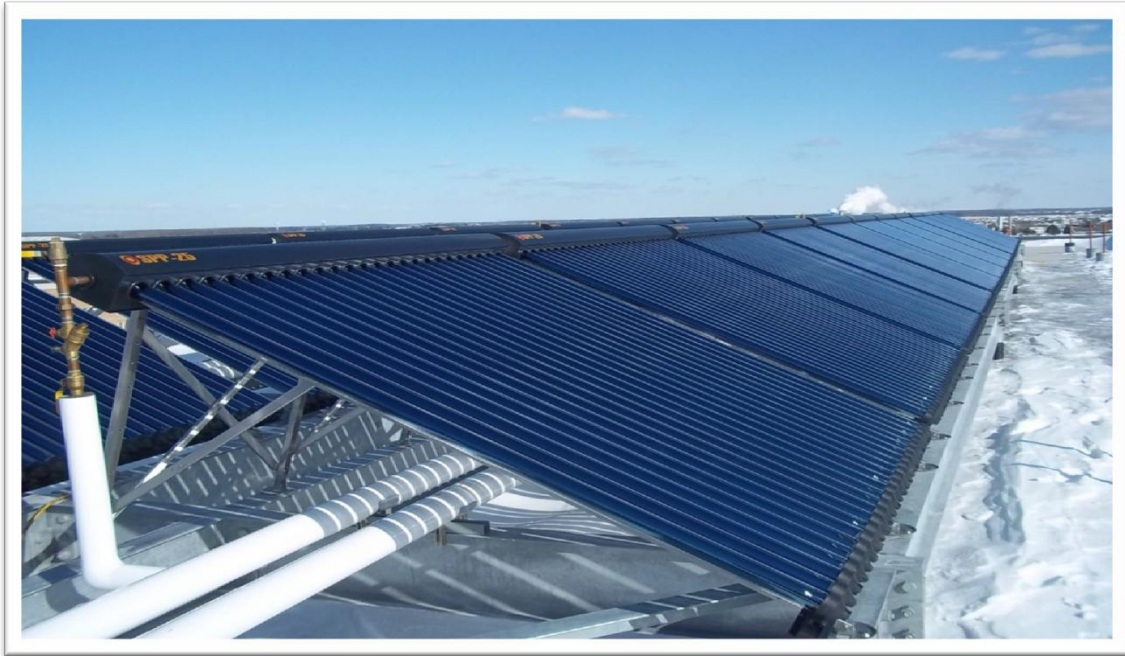
Solar thermo panels on the roof of the EHS Building
