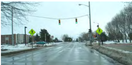
Broomfield Road at the pedestrian-activated traffic signal crossing.
