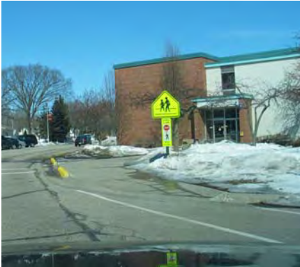
Example of existing pedestrian crossing signage on East Campus Drive.
