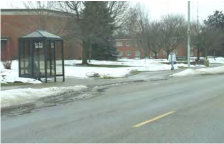
Bus shelter on northbound Washington Street, south of Anspach Hall.
