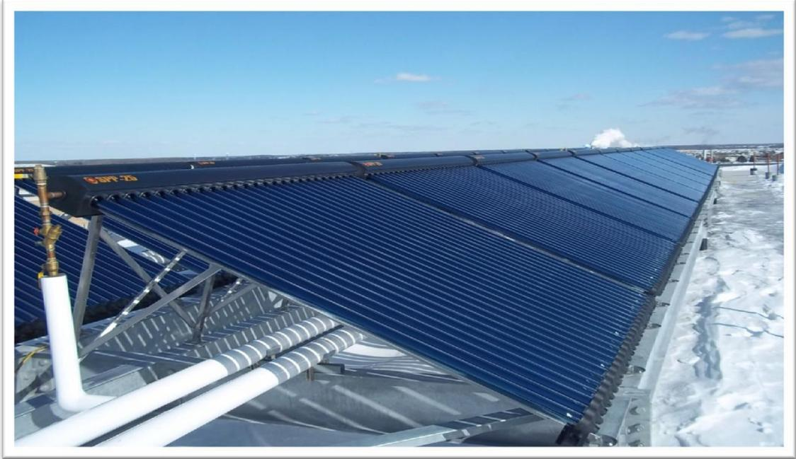
Evacuated Tube Solar panels on the Roof of the EHS Building
