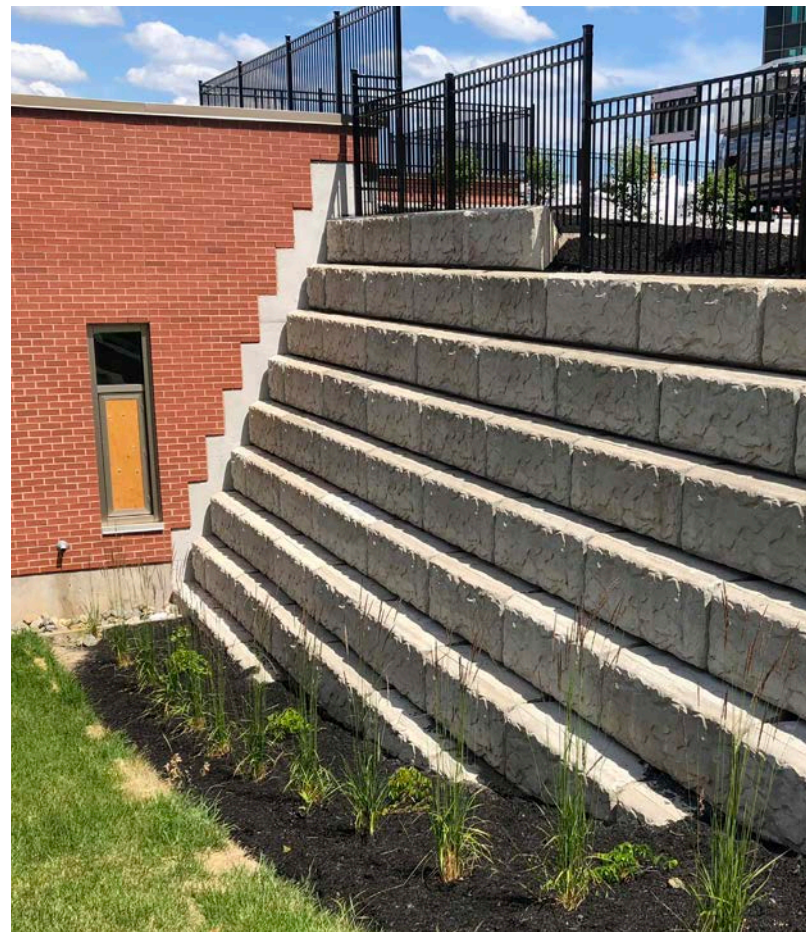
London Boulder Stone Retaining wall .
