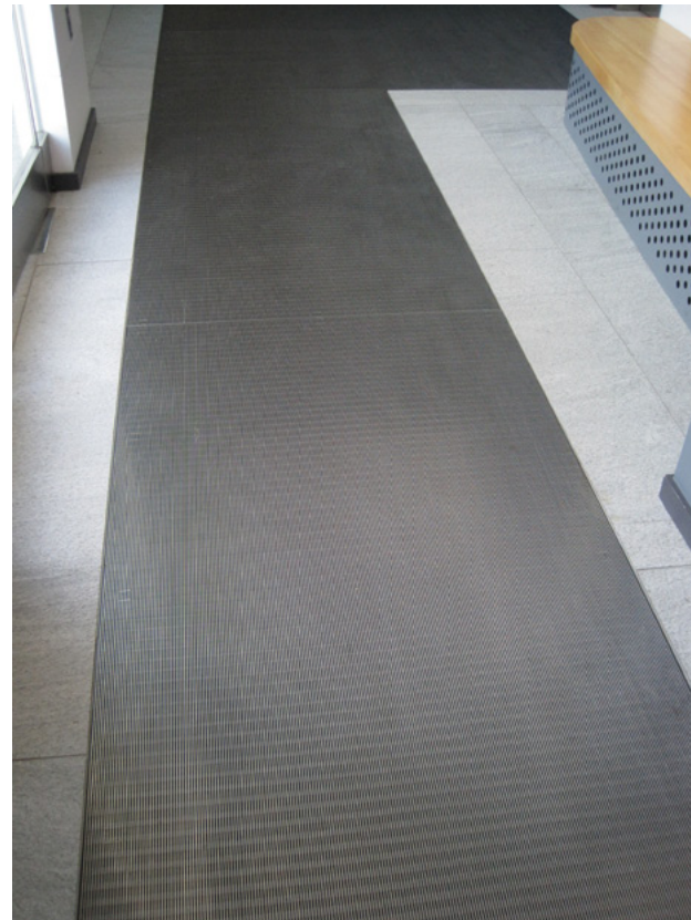
ENTRY GRATE, SKINNER HALL
