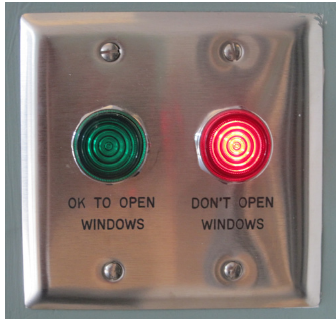
OPERABLE WINDOW INDICATOR, NORTH RESIDENTIAL DORM
