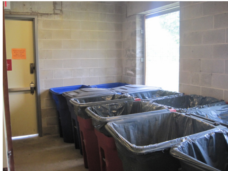
RECYCLING ROOM, NORTH D, NORTH RESIDENTIAL AREA
