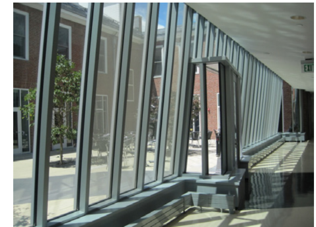
WESTERN GLAZING, SKINNER HALL
