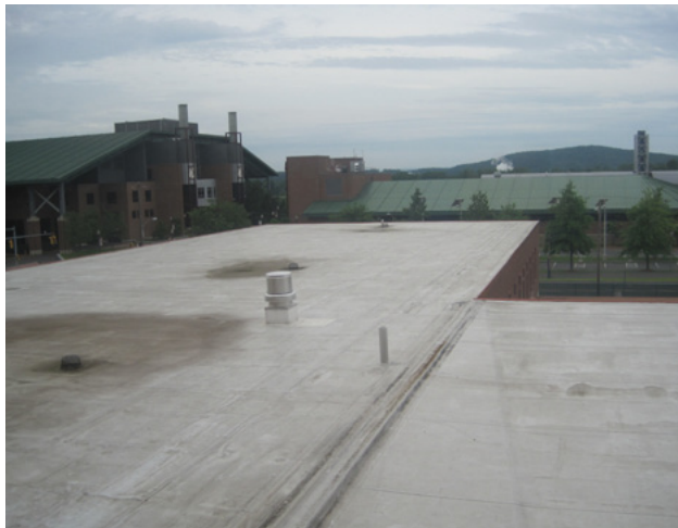
PHYSICAL PLANT ROOF, UMASS AMHERST
