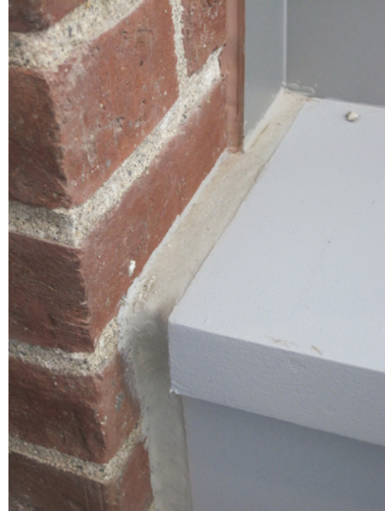
LOW VOC CAULKING, SKINNER HALL
