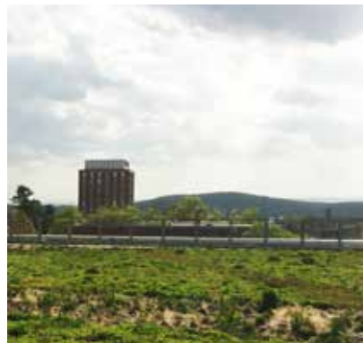
GREEN ROOF, INTEGRATIVE LEARNING CENTER, UMASS AMHERST
