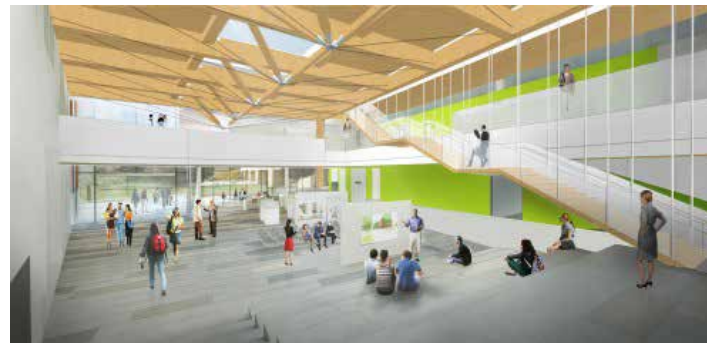
THE DESIGN BUILDING (SPRING 2017) HAS AN INNOVATIVE STRUCTURAL SYSTEM UTILIZING CROSS-LAMINATED TIMBER THAT WILL SERVE AS A LEARNING OPPORTUNITY FOR STUDENTS IN THE BUILDING AS WELL.
