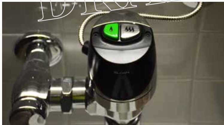
INTEGRATIVE LEARNING CENTER (2014) DUAL FLUSH TOILETS, UMass AMHERST
