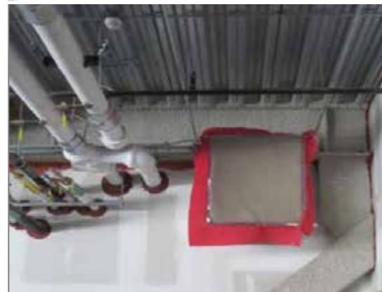
AIR HANDLERS MANAGE AIR QUALITY DURING CONSTRUCTION
