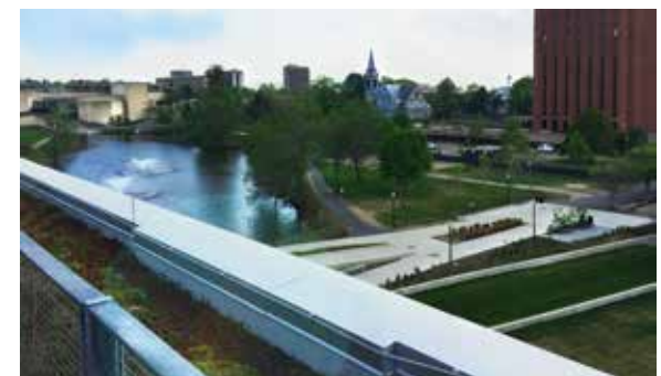
LIGHT COLORED WALKWAYS HAVE A LOW SRI. PHOTO TAKEN FROM ILC ROOFTOP
