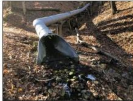
Outfall of Au Sable pipe system at toe of ravine
