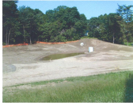
Under construction - May 2001
