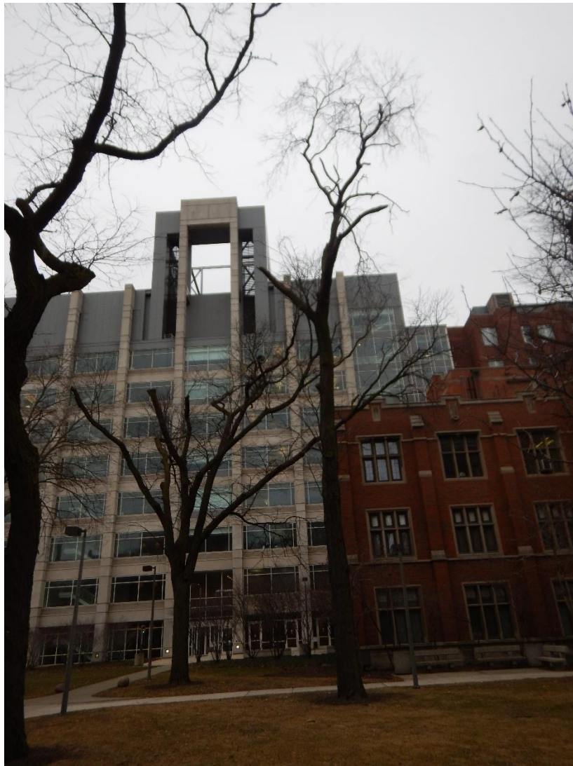
Trees #3685 (right) and 3705 (left) recommended for removal because of major dieback.
