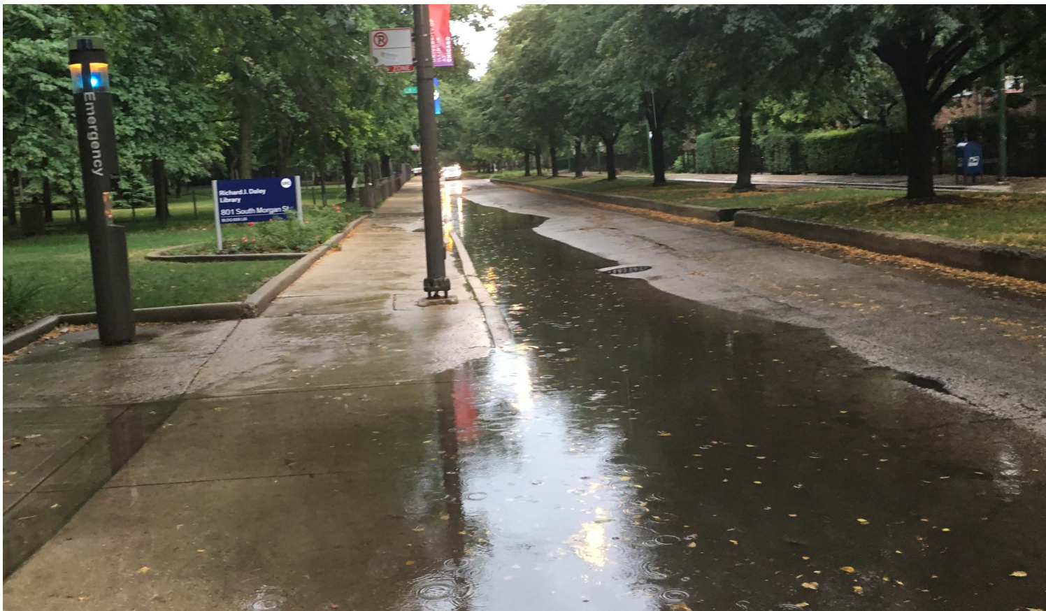
Photo: Stormwater from a heavy rain event in 2017 floods not only City-owned streets, but also UIC property like sidewalks such as this one near the entrance of the Daley Library.
