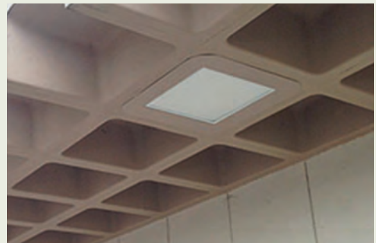
CSU Dominguez Hills LED lighting
