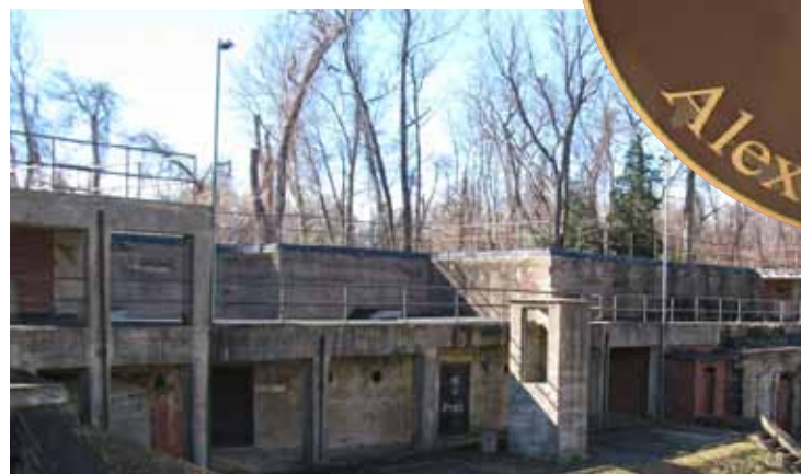
Mt. Vernon Battery gun emplacement site in Ft. Hunt Park was built for the Spanish American War.
