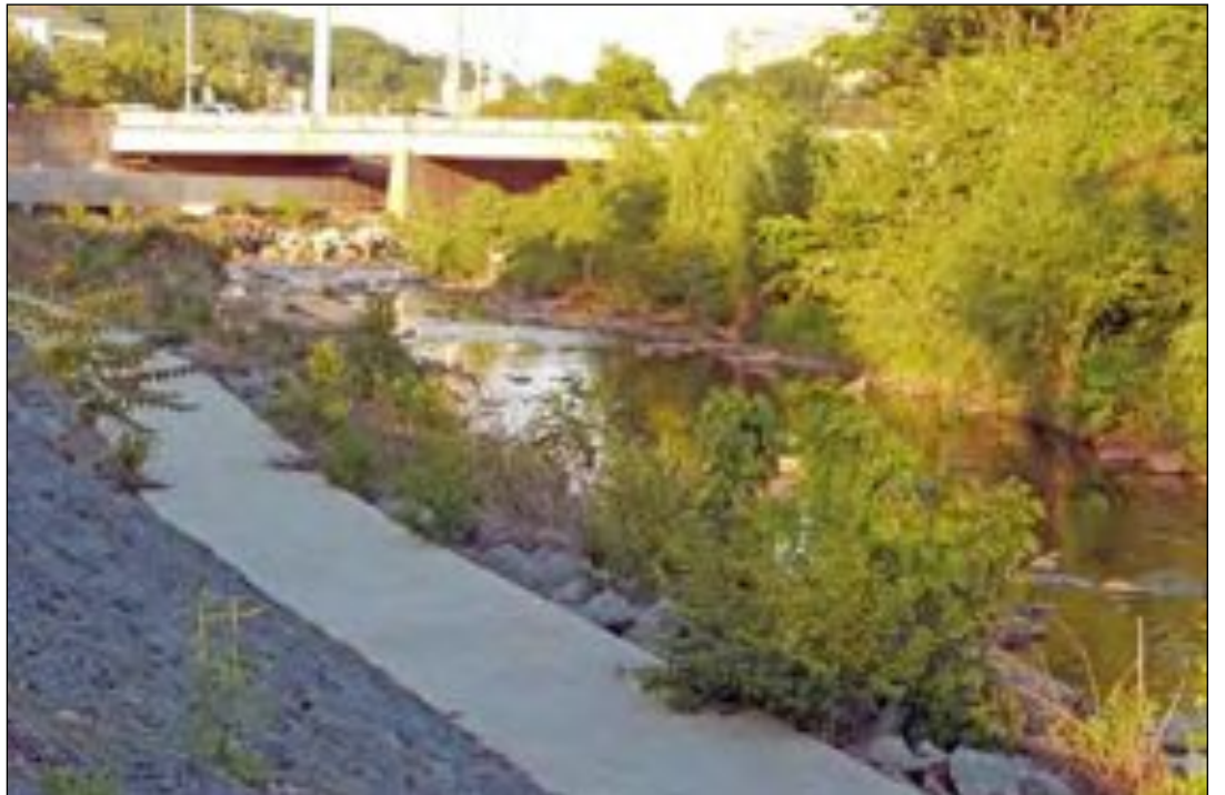
Four Mile Run, looking towards West Glebe Road.
