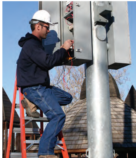
Having major electrical components accessible at ground level avoids hiring a $100/hour crane to replace a $10 fuse.
