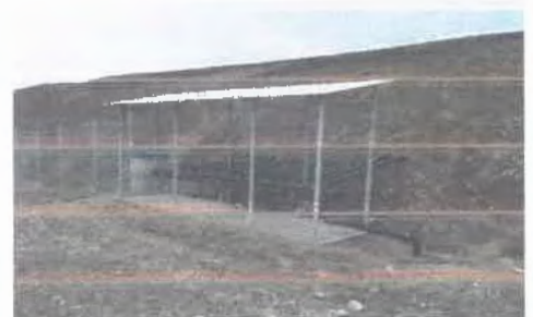
Conducte colectare biogaz
