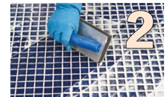
Remove excess ARDEX EG 8 PLUS from the surface
