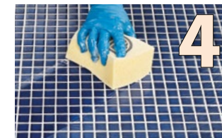
Clean down the tile surface to remove emulsified residues
