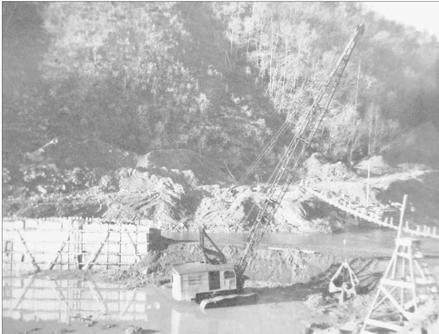
Above, Philpott Dam construction begins to control the Smith River.
