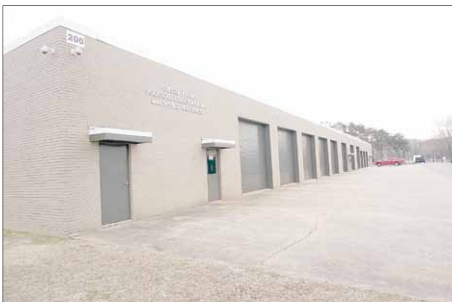
Part of the Chester R. Lane Vocational Educational Building on the MHS campus has been redone for the robotics program. The building previously housed auto body classes.
